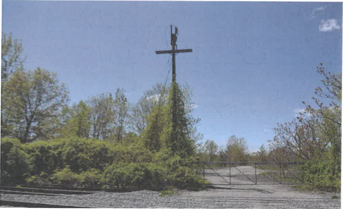
03. SW Quadrant and Old Electrical Pole
